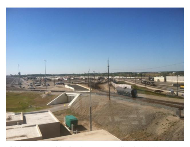
This is looking west from the brand new hump control tower. The tank car is heading for the working original half of the yard with all those cars in the distance. The new class yard extending out of the frame on the left effectively doubles the size of the "bowl" and the tank car is atop the double crossover that will allow cars from either of the two hump tracks reach any track in the bowl. That's how you double the number of outbound train-starts.
