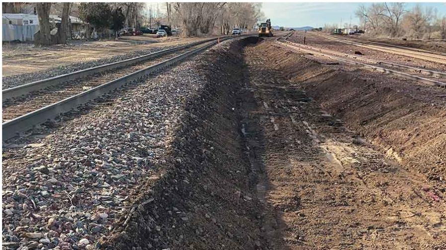
This track bed excavation is for a siding extension project on the Phoenix line at Ash Fork, Arizona, just south of the Williams junction on the ex-Santa Fe transcon. Genesee & Wyoming’s Arizona & California short line, winner of the BNSF Short line of the Year award, joins the Phoenix line at Wickenburg.
